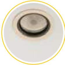
1. Old recessed ceiling light with a larger ceiling cut-out
