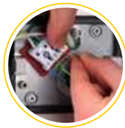
Connection of the power line
